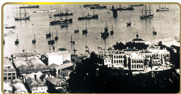
The Seamen's Hospital under renovation and reconstruction in 1873.
